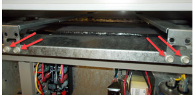
FIGURE 6 Remove Four Screws
