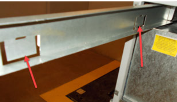
FIGURE 5 Bend Filter Tabs Down
