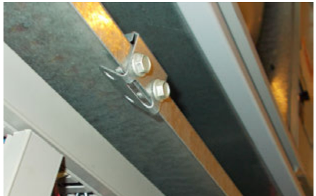
FIGURE 8 Re-Install Screws and Bend Tabs Up
