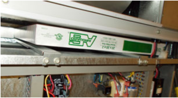
FIGURE 10 Install Left 2" Filter
