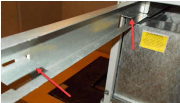
FIGURE 4 Filter Tabs in Up Position
