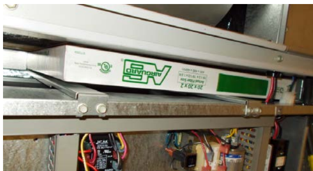
FIGURE 10 Install Left 2" Filter
