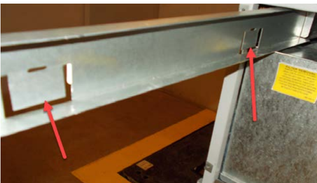
FIGURE 5 Bend Filter Tabs Down
