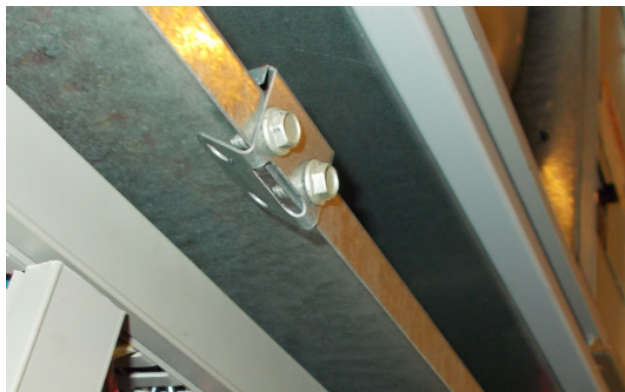
FIGURE 8 Re-Install Screws and Bend Tabs Up
