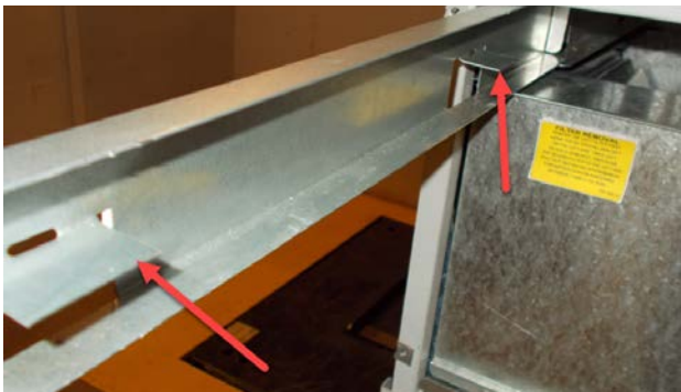
FIGURE 4 Filter Tabs in Up Position
