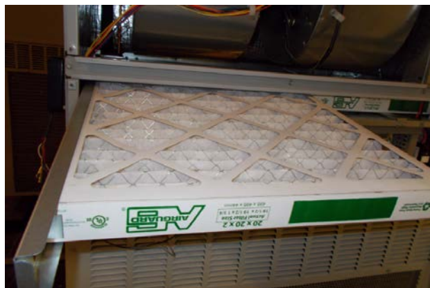
FIGURE 10 Install Left 2" Filter
