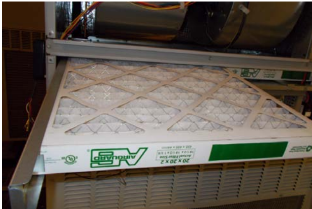
FIGURE 10 Install Left 2" Filter
