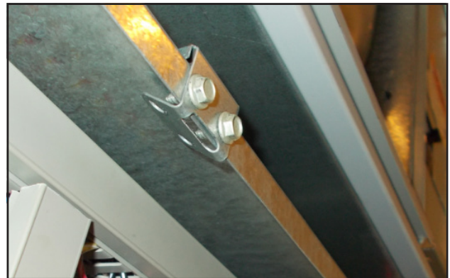
FIGURE 8 Re-Install Screws and Bend Tabs Up
