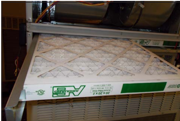
FIGURE 10 Install Left 2" Filter
