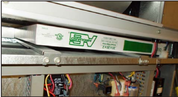
FIGURE 10 Install Left 2" Filter
