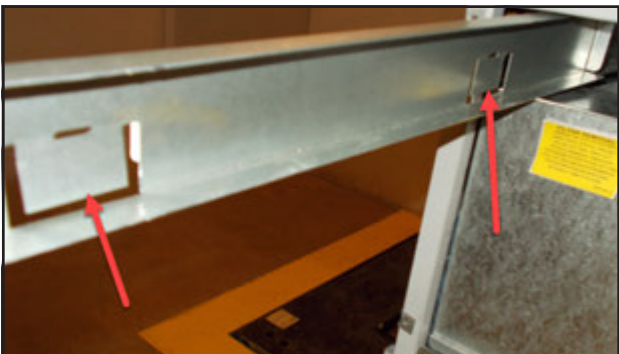
FIGURE 5 Bend Filter Tabs Down
