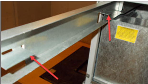
FIGURE 4 Filter Tabs in Up Position
