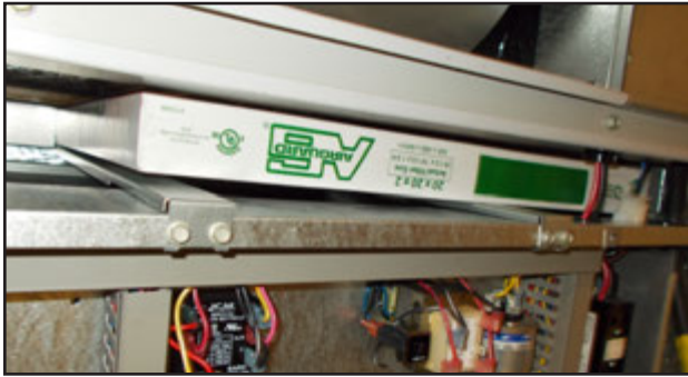
FIGURE 10 Install Left 2" Filter
