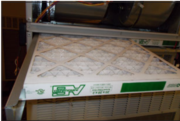
FIGURE 10 Install Left 2" Filter
