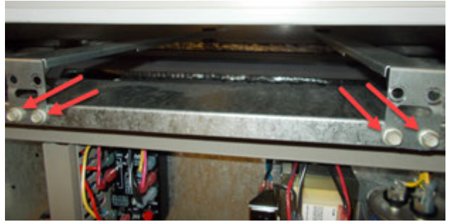
FIGURE 6 Remove Four Screws
