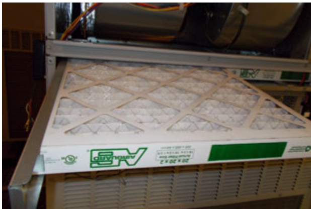
FIGURE 10 Install Left 2" Filter
