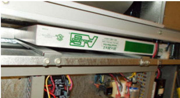
FIGURE 10 Install Left 2" Filter
