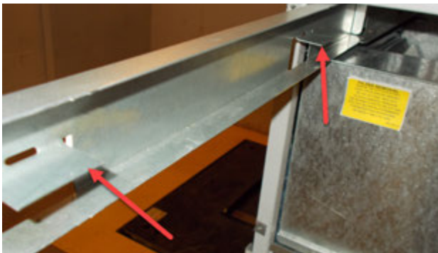
FIGURE 4 Filter Tabs in Up Position
