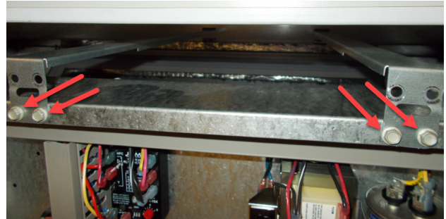
FIGURE 6 Remove Four Screws
