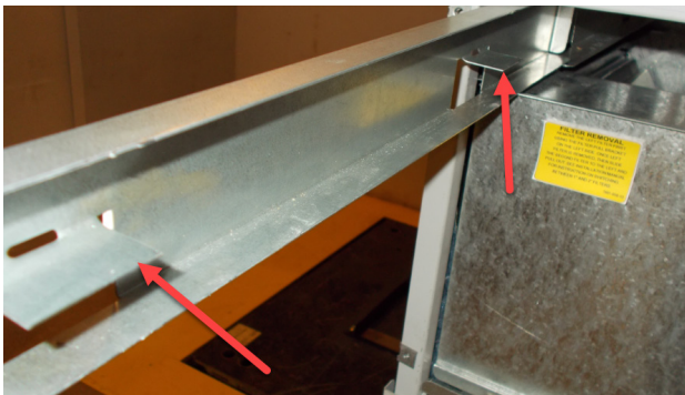
FIGURE 4 Filter Tabs in Up Position
