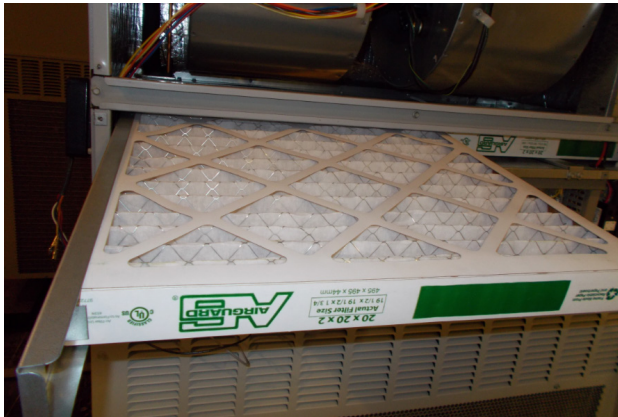
FIGURE 10 Install Left 2" Filter
