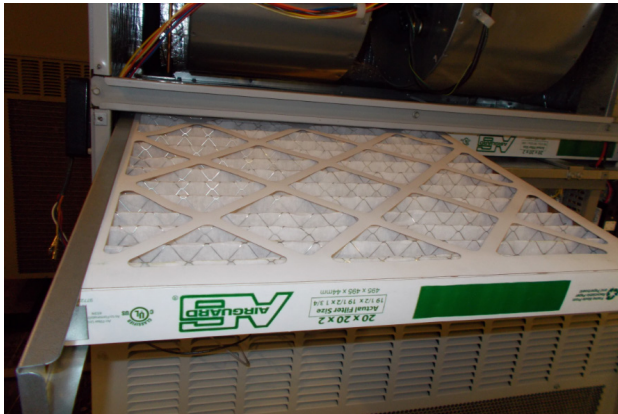
FIGURE 10 Install Left 2" Filter
