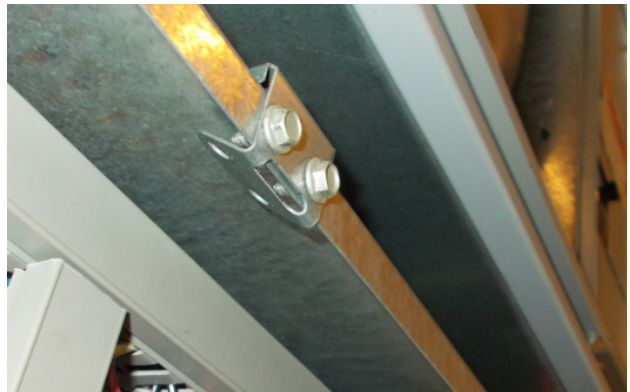
FIGURE 8 Re-Install Screws and Bend Tabs Up
